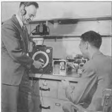
FIGURE 15. A. P. G. Peterson (right) and R. J. Ruplenas with an experimental u-h-f signal generator.
