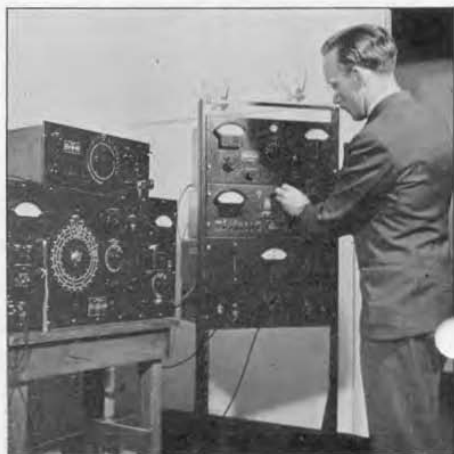
FIGURE 11. C. A. Cady, of the Audio-Frequency Group, checks the distortion in a newly-developed oscillator.
